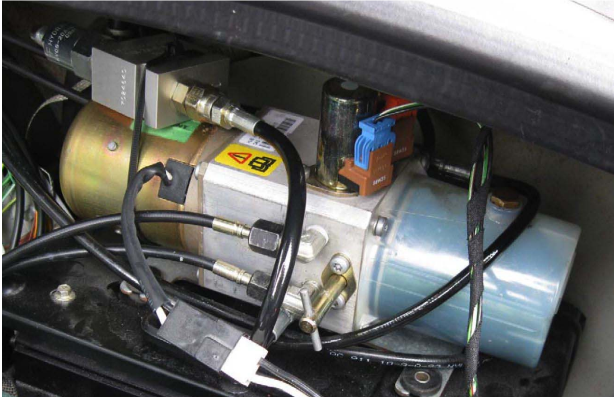
Figure 5 – Pump and kit installed
