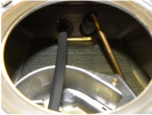
View into tank showing two fuel lines coming into tank.
